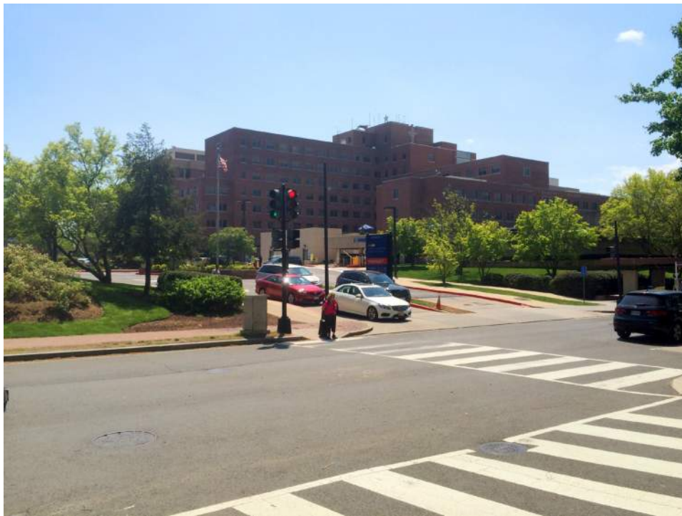
5. VIEW FROM RESERVOIR RD & 38TH ST
